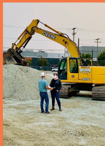
Jen at the construction site.
